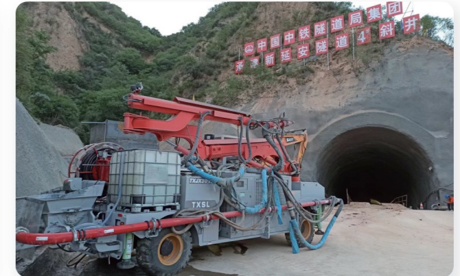
延安隧道4#斜井 Yan'an Tunnel 4 # inclined shaft
